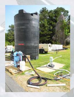
Injection of the Bioaugmentation Culture into surficial groundwater wells to accelerate biodegradation of VOCs
