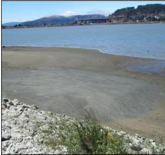
Leachate area with clay mat in place
