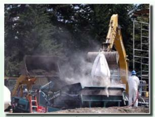
At the former Evergreen Infiltration Range, a phosphate-based stabilizer is added to prevent lead in the soil from leaching during a soil recycling project.
