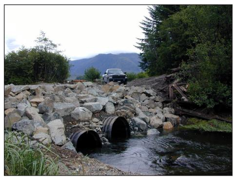
▲ To access certain sites today, the construction of roads was necessary. This access road was constructed across a salmon stream, requiring timing and specialized engineering to minimize impacts to spawning salmon. Courtesy of USACE/Jacobs.
