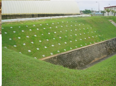
Before and after photos of the benefits of soil-nailing technology on Camp Hansen.
