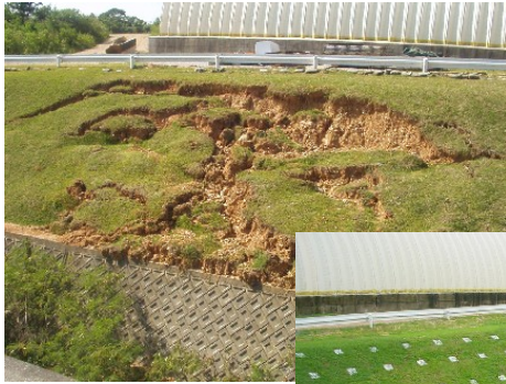
Before and after photos of the benefits of soil-nailing technology on Camp Hansen.
