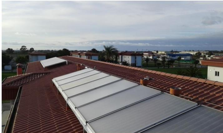
Figure 4: Solar Thermal Panels installed on 13 barracks roofs for hot water heating providing 13,402 MBTU/year in energy savings.
