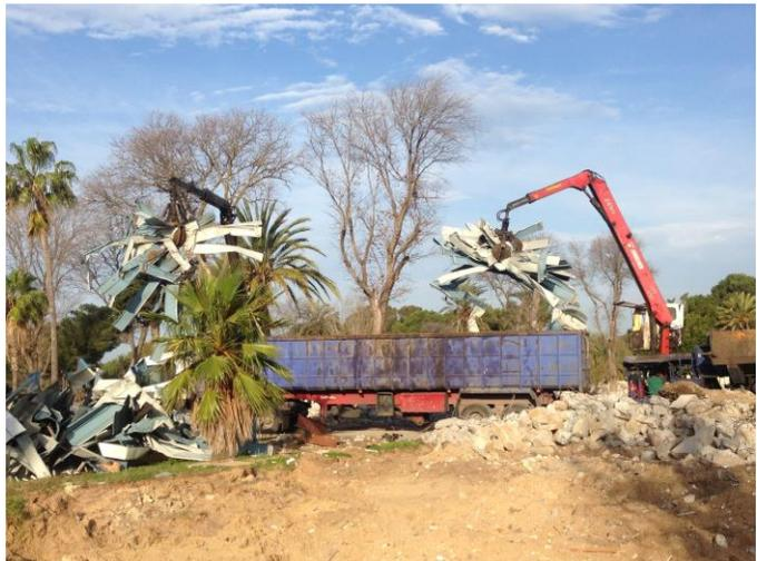
Figure 3: Recycling contractor compacting material on site, reducing transportation costs and increasing profit for the government.
