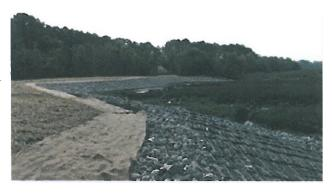
steel frame was used to support the mesh when filling each of the mattresses with a front end loader. The mattresses were placed, utilizing heavy equipment, so the toe of the mattress was at 4-ft elevation and the head was at about 12-ft elevation. More than 850 tons of Class A riprap was used to fill the 110 marine mattresses needed to protect the 500 feet of shoreline.
