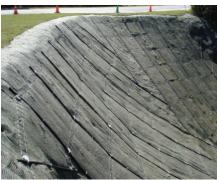
The failed slope near Classroom 1 at the JWTC was effectively stabilized with the use of soil nailing and vegetation matting.
