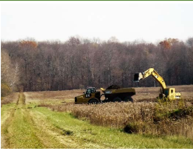
This up-armored excavator is loading contaminated soil into the dump truck which will transport the soil to the munitions screening area at Winklepeck Burning Grounds during the 2016 Remedial Action.
