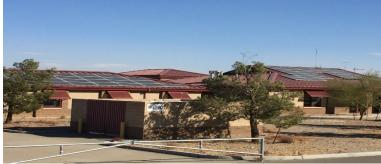
The Bachelor Enlisted Quarters has 75 kW of solar photovoltaic panels installed on the roof of the building as the nearby carport.
