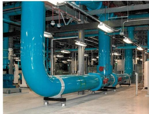
*The NSA's chilled water distribution system keeps high performing computer systems cool and functional, allowing critical intelligence community missions across the globe to proceed without impediments. These chilled water pipes are located in the high-performance computing center.*
