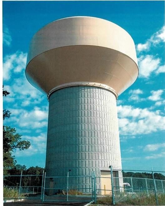
*Pictured here, a 1-million-gallon storage tank located on NSA's main campus stores reclaimed water for cooling facilities and infrastructure on NSA's East Campus.*
