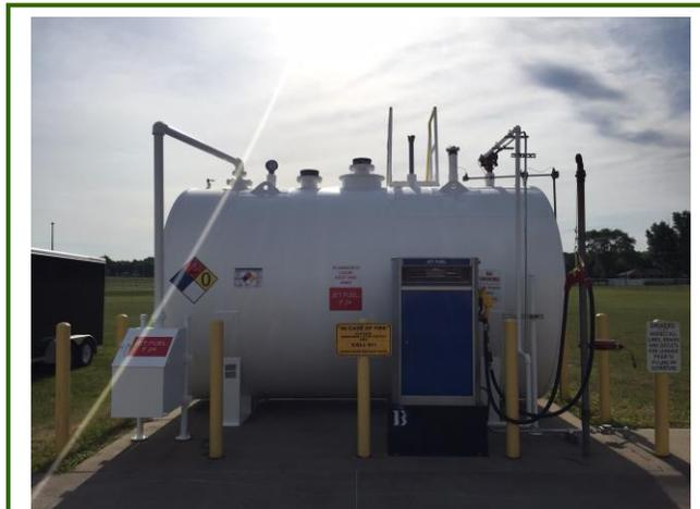
WIARNG Fueling System Upgrade project. Picture depicting upgraded above ground storage tank with new dispenser and leak detection along with system connected to WIARNG Federal network for remote access. Below, new fueling system tank monitoring panel.
