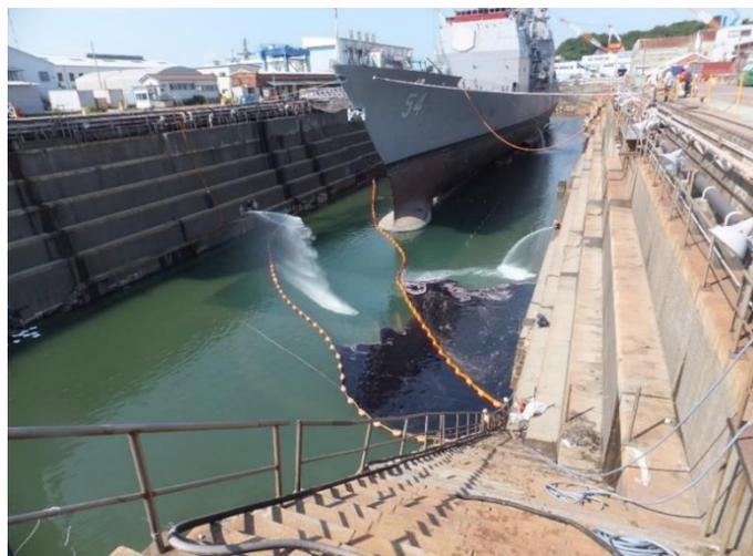
170617-N-YU361-017 Floating harbor booms provide excellent containment and control of oil for rapid recovery during the docking of USS ANTIETAM (CG 54). SRF-JRMC oil spill management team members from Commander Fleet Activities Yokosuka Port Operations pre-staged the booms.
