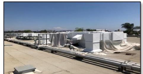
**Chemical protective coatings applied to HVAC units reduce the need for maintenance and replacement, and help the equipment operate more efficiently.**
