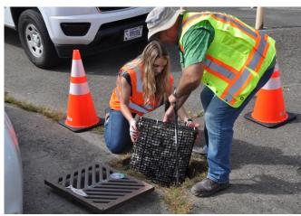
Chris Jorgensen and Kelsey Hall, two environmental engineers within the NAVBASE Kitsap's Environmental Division, deploy crates of oyster shells. Zinc concentrations in the stormwater system of NAVBASE Kitsap Keyport are effectively lowered by deploying the shells.
