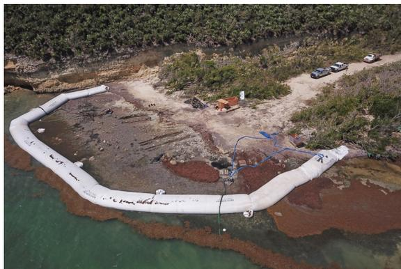
*Innovative use of a temporary, water-filled cofferdam significantly enhanced the safety and efficiency of operations to remove munitions located just offshore. The cofferdam allowed the site to be dewatered, such that UXO technicians successfully removed munitions without the need for UXO divers, thus accelerating the cleanup while increasing the safety of the operation.*
