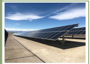
A newly installed photovoltaic solar system on Colorado's Fort Lupton Readiness Center absorbs and converts solar energy, July 2020. The Colorado Department of Public Health and Environment's Supplemental Environmental Program funded the 150kW Photovoltaic Solar array at the Fort Lupton Readiness Center in Colorado. Electricity generated by the solar panels will offset 100% of the facility needs which makes the Readiness Center Net-Zero electric.
