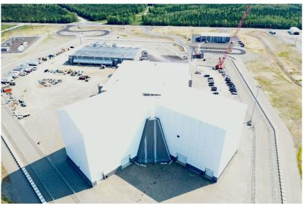
Photo 1 - Aerial photograph of the Long Range Discrimination Radar (LRDR) at Clear Space Force Station, Alaska, July 19, 2019. Temporary structures provide protection during radar installation and integration.
