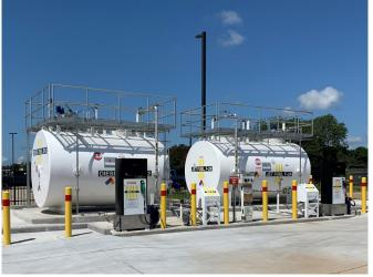
Two newly installed ASTs that replaced three aging USTs in the Aerospace Ground Equipment yard.
