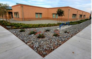
Erosion control at the Seal Beach Reserve Center. The installation installed multiple retention basins and LIDs to ensure building and surface runoff is captured before draining into adjacent channels leading to the Anaheim Bay.
