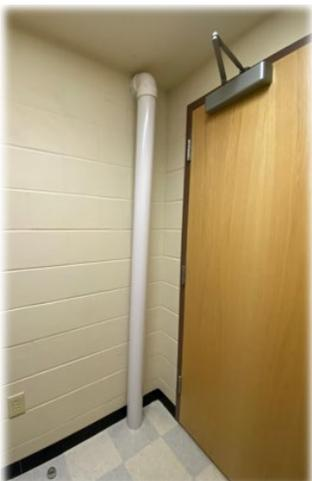
Radon Reduction System installed in Storage Room, Building 214
