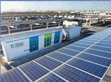
The MCAS Miramar hosts a 100% renewable microgrid that can support over 100 mission-critical facilities for three weeks if disconnected from the grid. The microgrid integrates battery storage, controllable photovoltaic, electric vehicles, and complete load management within
