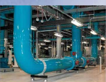
The NSA's chilled water distribution system keeps high performing computer systems cool and functional, allowing critical intelligence community missions across the globe to proceed without
