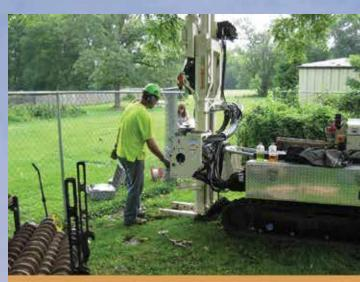
Staff install a groundwater monitoring well in Waupun, WI, for in-house spill cleanup site investigations. The installation achieved complete closure of the site in May 2018, and personnel eliminated offsite impacts to avoid groundwater use restrictions on adjacent properties.
