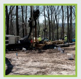
Department of the Air Force environmental restoration contractors drill a small-diameter pipe into the ground at Sans Souci Farm in Sumter, South Carolina, to inject a Remediation Products BOS 100 treatment into a deep trichloroethene/ tetrachloroethene plume. This technique intercepts and treats the plume's leading edge.
