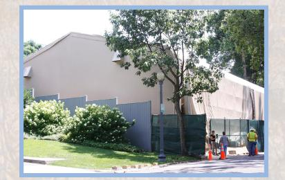
A tent covering the Glenbrook Road Remedial Action site enabled safe, efficient work. The team remediated, removed, or recovered 556 munition items, 2,139 pounds of laboratory debris, 53 intact and sealed glass containers of chemical agent, and 7,500 tons of contaminated soil.
