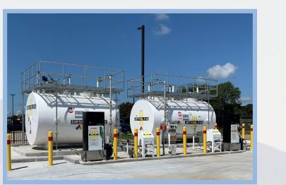
Two newly installed above-ground storage tanks (ASTs) replaced three aging underground storage tanks (USTs) in the Aerospace Ground Equipment yard. The two environmentally safer AST systems replaced UST capacity of 48,000 gallons with only 11,000 gallons of above-ground storage.
