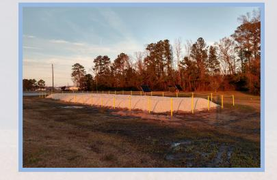
In FY 2020-21, MCB Camp Lejeune evaluated alternative treatment technologies across sites to address contaminated groundwater and expedite site closure. This subgrade biogeochemical reactor treated about 93,000 gallons of groundwater at Installation Restoration Program
