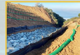
Site restoration in the steep ravine after excavation of solid waste debris and contaminated soil was completed at IR Site 7. Photograph depicts stormwater channel riprap and erosion controls.
