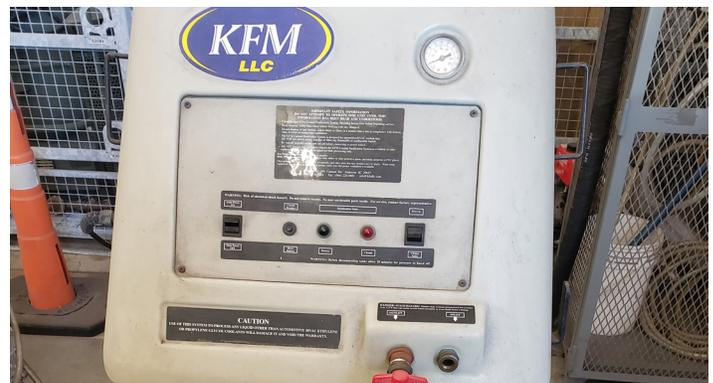
KFM, LLC coolant purification system used to recycle used antifreeze at MCSF-BI. Used antifreeze is collected by shop personnel and transferred into a used anti-freeze tank at Building 350. Once a sufficient volume has been collected, it is processed through the coolant purification system and transferred into a purified anti-freeze tank for dispensing to shops.
