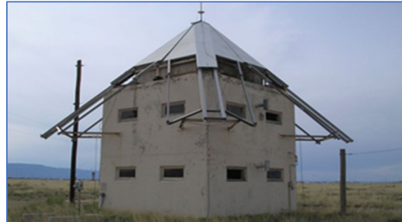
Cold War Missile-Tracking Tower Early Cold War cinetheodolite missile-tracking tower. These structures were built to track missiles during the early phases of the post WWII period.
