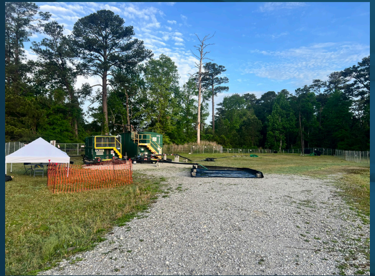
Site 88 Zone 2 potassium permanganate injection layout, including tanks to store permanganate solution and recirculation water and distribution piping connecting to the well heads.
