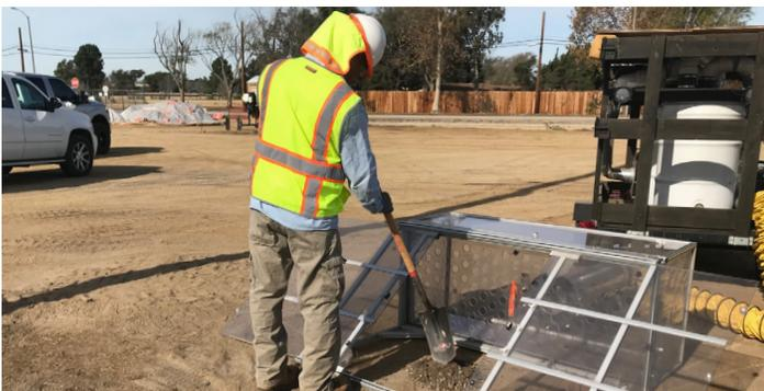
*The NBVC Environmental Restoration Program developed an innovative mobile chemical agent containment hood at the former GMTA to remediate CAIS containing phosgene, chloropicrin, mustard gas, and lewisite. Using this negative pressure device protects residents in nearby military family housing and workers at the site.*
