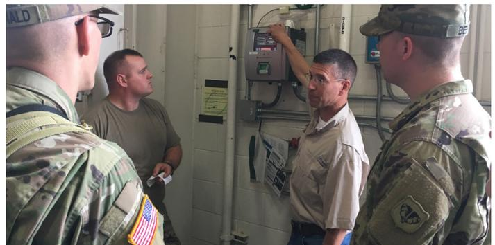
Mr. Scott Rickard, Construction and Facilities Management Office-Environment, trains soldiers to operate a new tank monitoring panel connected to a fueling system. The panel is remotely connected into the Federal network for remote access and efficient management.
