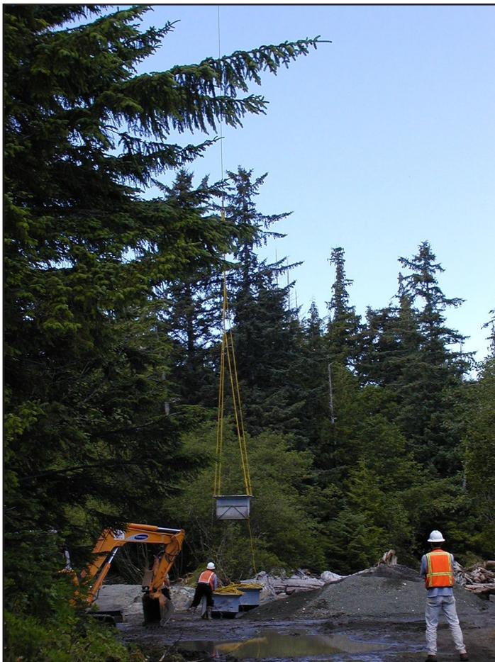
▲ In some cases, helicopter transport of contaminated and backfill material was more economical and less environmentally damaging when compared to the construction of access roads. Courtesy of USACE/Jacobs.
