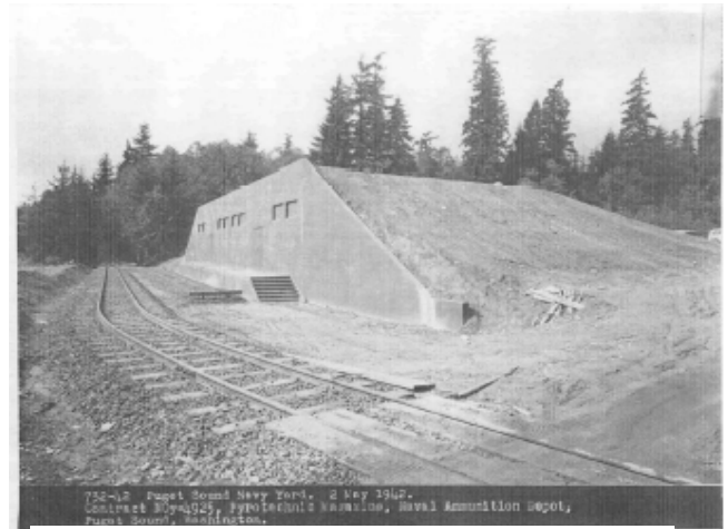
Explosives magazine at former Puget Sound Naval Ammunition Depot (now site of Jackson Park Housing). 1942.
