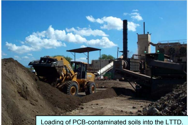
Loading of PCB-contaminated soils into the LTTD.
