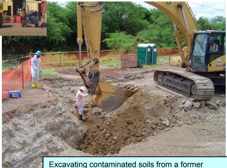
Excavating contaminated soils from a former transformer site.
