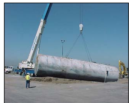
Underground storage tank removal.
