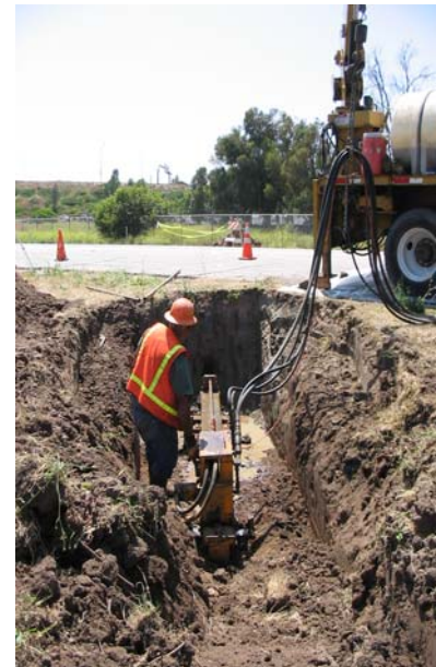
Shallow Groundwater Unit Cleanup - Site 24 Horizontal Boring
