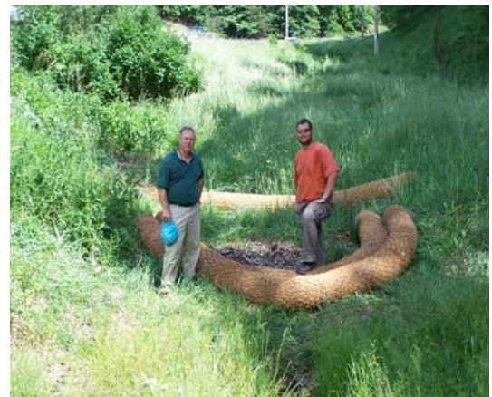
Installation of Bio-logs at the Operations Site
