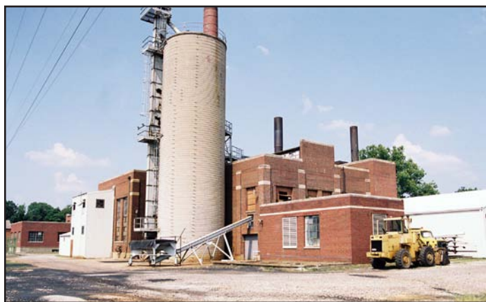
The Muscatatuck site has its own power plant, pictured above.
