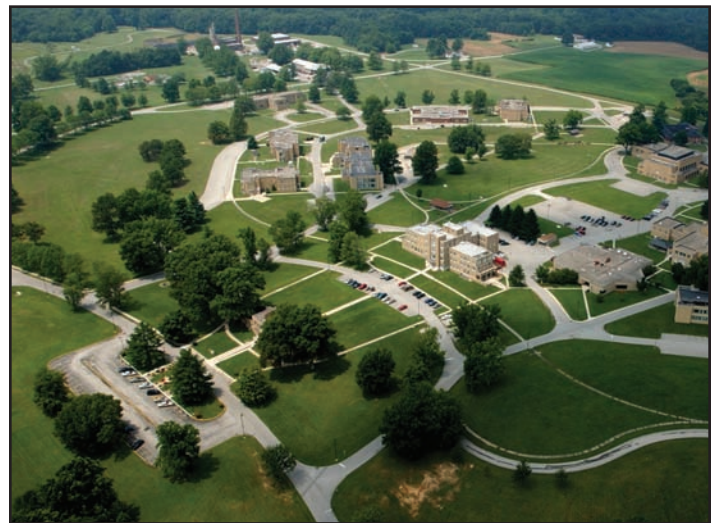
Aerial photograph of some of the buildings on the Muscatatuck Urban Training Center.
