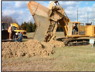
*The barrier was installed using a one-pass trench excavator, which simultaneously excavates soil and emplaces the barrier's reactive material.*
