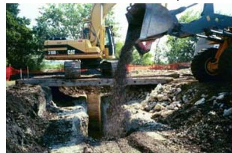
**Photo 4** Media backfilling
