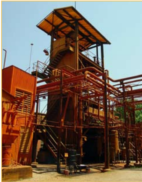
Part of the World War II carbonyl iron plant in the Carbonyl Iron Unit Historic District at Redstone Arsenal. This is one of only three known active carbonyl iron plants in the world. The district has undergone very little modification since it first began production in 1943.
