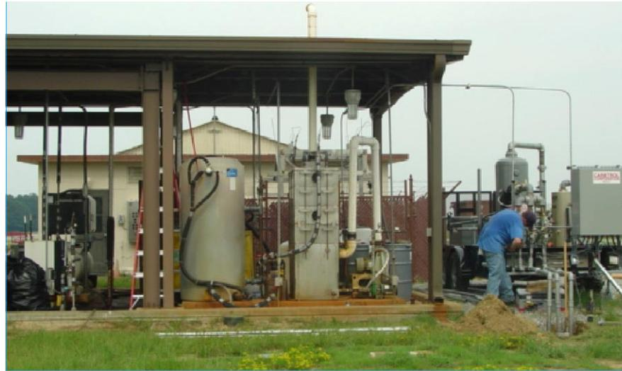
Multi-phase extraction system treating fuel contamination at a hydrant spill site.
