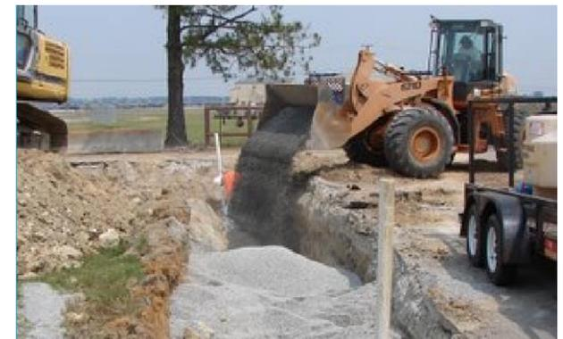
Construction of interception trench for in-situ bio-augmentation treatment at the Old Jet Engine Test Cell site.
