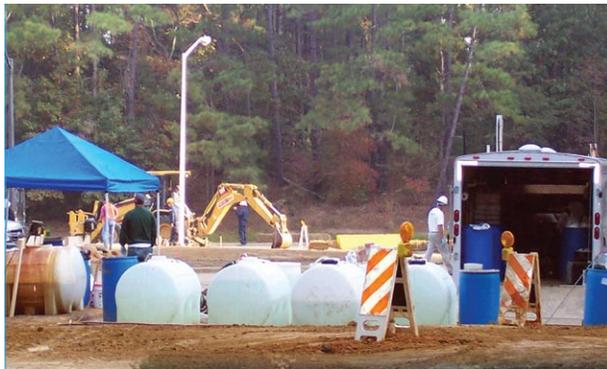
Injection of Fenton's reagent oxidant/catalyst reduced groundwater contamination.
