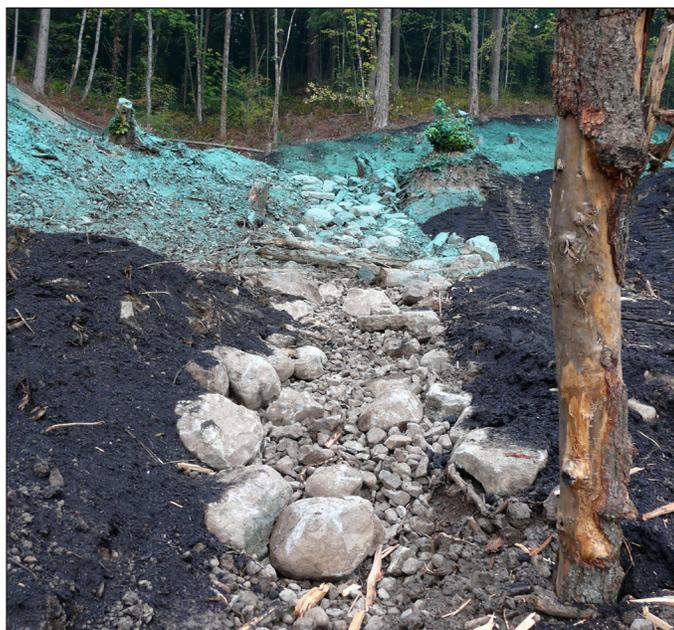
Habitat reconstruction began during the restoration phase. Hydroseeding with native grass species, applying biodegradable geotextile materials, and irrigating with water recycled from the soil treatment system facilitated erosion control and laid the groundwork for this area's future use as hiking and biking trails.
