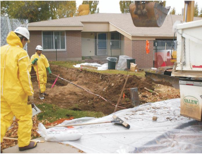
A large-scale PCB cleanup in a base housing area was completed in just 22 months and hauled away 63,000 cubic feet of contaminated soil.
