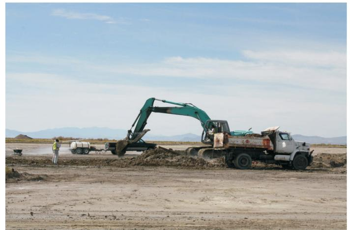
Construction contractors excavate an on-site landfill at Wendover Air Force Auxiliary Field, into which 4,200 cubic yards of asbestos-containing materials and contaminated soil would be placed. Landfilling the material on-site saved the Air Force nearly \$1 million in transportation and disposal costs.
