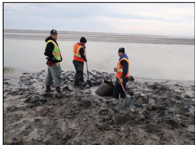
Photo 1. Sam Widmer (left) with Weston Solutions works with Eric Jenks (center), and Mike Flisk (right) with Marsh Creek, LLC to retrieve a buried drum from a sand bar in the Jago River delta. Over 1,400 drums were recovered from the Jago River area.
