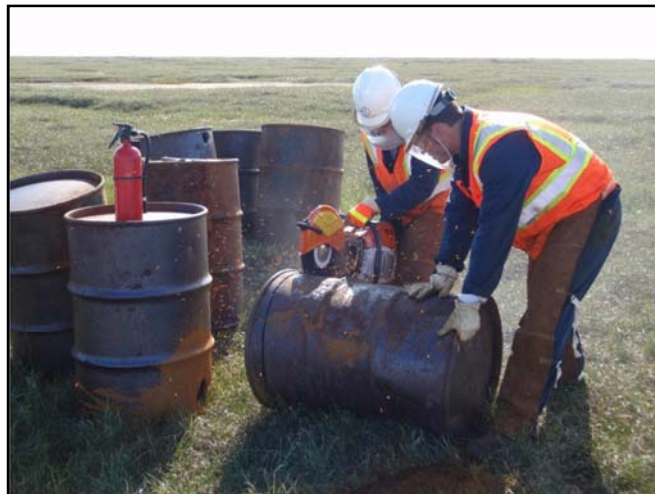
Photo 3. Darren Kayotuk (left) and Eric Jenks (right) utilize a demolition saw to dehead a drum before cleaning out residue inside.
