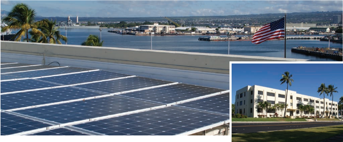
Building 150, a 1940 historic building at Joint Base Pearl Harbor-Hickam (JBPHH), and headquarters to both Commander Navy Region Hawaii and Commander JBPHH, is one of five structures at Pearl Harbor that is part of a $15 million Photovoltaic (PV) panel project. Four hundred sixty two, 235 watt PV panels have been installed on the roof with an anticipated production of 108.57 kilowatts at its peak output.
