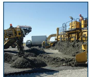
In 2010/2011 Fairchild completed a major reconstruction of the runway. In total, an incredible 90,000 tons of concrete, 106,000 tons of asphalt, and 125 tons of metal were salvaged, recycled, or reused. In addition, \$12 million dollars of new concrete used on the runway contained recycled fly ash as a component.
