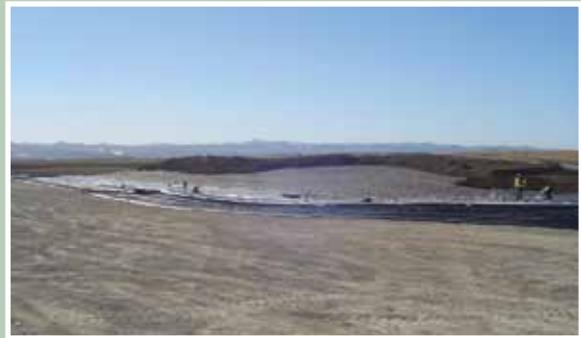
*MINS installed the IA-H1 landfill cap over the Containment Area covering approximately 73 acres of the IA-H1 site. The gentle sloping of the cap design decreases potential erosion and thus decreases maintenance costs. In this photo, the field team is installing the geo-composite venting layer.*
