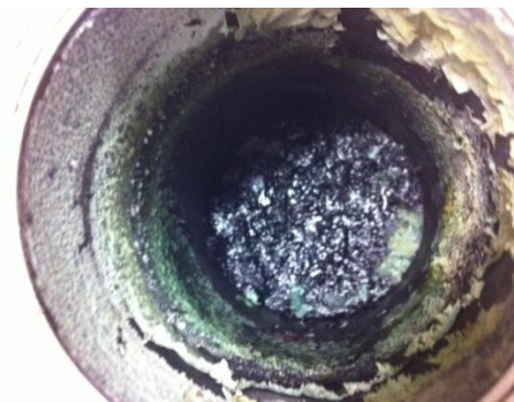
Photo 3 - Corroded laboratory vessel from reactions of counterfeit refrigerant with air conditioning system materials.
