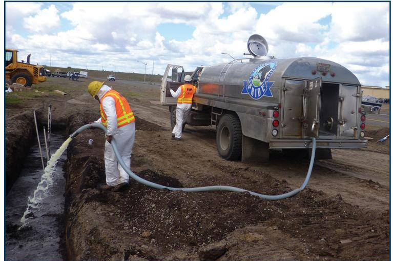
Cheese whey being applied during the construction of the sustainable bioreactor demonstration project. Fairchild AFB worked cooperatively with a local creamery to enable the reuse of cheese whey, a bi-product from creamery processes. The cheese whey served as a necessary carbon source within the construction of the solar-operated bioreactor and promotes the breakdown of contaminants in groundwater using natural processes.
