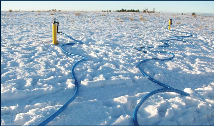
Dual-purpose remediation wells are connected to the soil vapor extraction system. Soil vapor extraction has been implemented in conjunction with in-situ chemical oxidation injections, and batch operations at the existing groundwater extraction and treatment system. The triad of remedies implemented has optimized chlorinated solvent removal and degradation at Craig Road Landfill.
