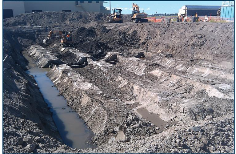
Removal projects performed at two former underground storage tank sites. These projects were strategically executed during a runway replacement project, and resulted in no mission impacts. The removal actions resulted in the removal of 12,000 tons of contaminated soil and concrete, and the treatment of 310,300 gallons of contaminated groundwater.
