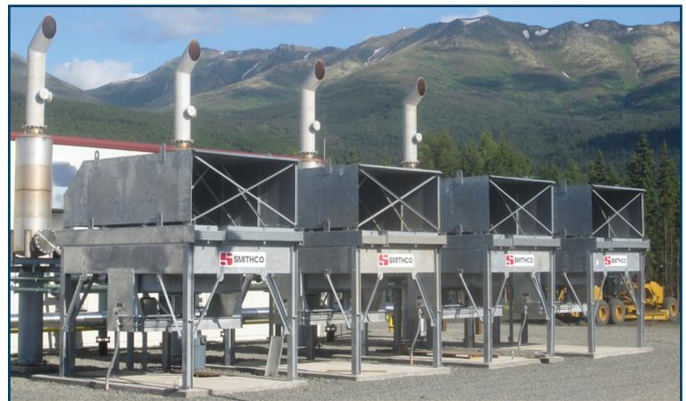
The JBER Landfill Gas Waste-to-Energy Plant was constructed with 4 generator units designed to run on methane gas that is produced by the breakdown of wastes buried in the landfill. A 5th generator unit is expected to come on line in 2013, producing 26.2 % of JBER's electrical load.
