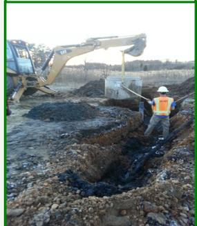
Hydraulic Containment: extraction wells and injection wells connect via buried lines. A similar process is used for air sparging and vapor extraction.
