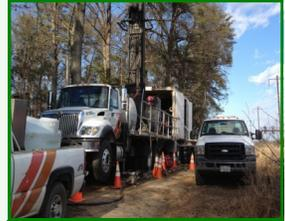
Rotosonic drilling for monitoring well installation
