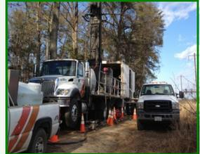
Rotosonic drilling for monitoring well installation
